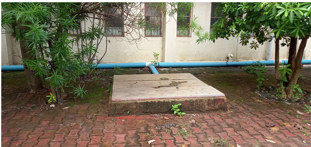
Rain water harvesting pit
